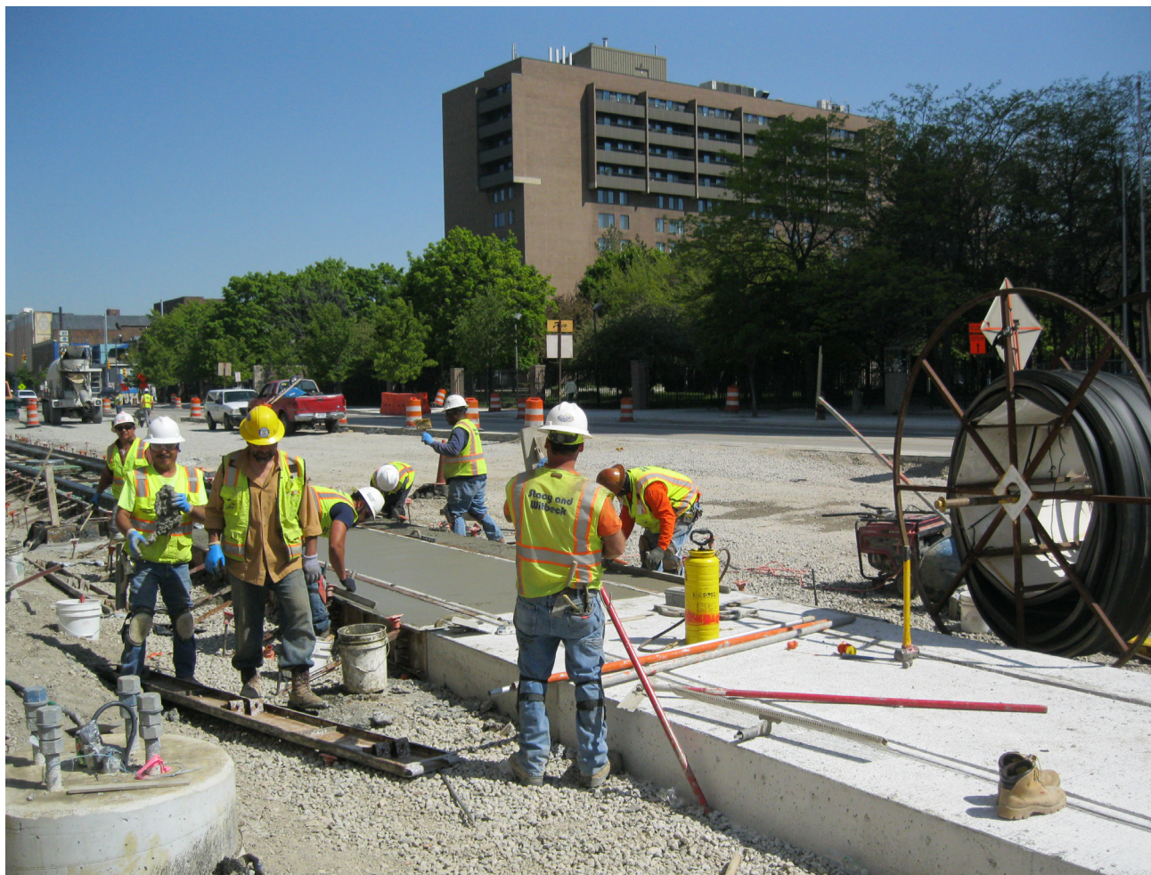
Above: The RTA's current and future goals include the construction of additional rail lines to serve the region.
